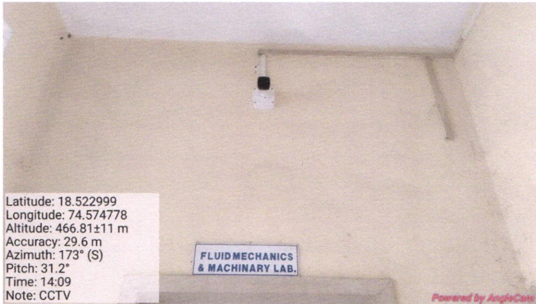
Photo of CCTV
