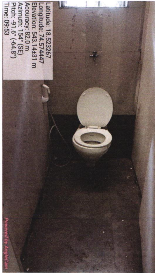
Photo of Divyangjan Friendly Washroom
