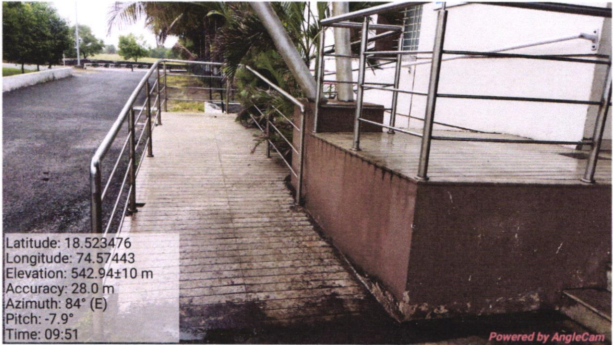
Photo of Ramps for Divyang
